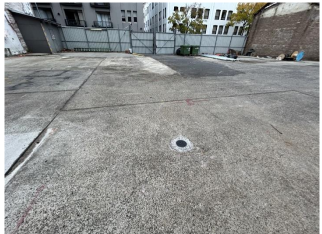
Figure 31 View north detailing a ground monitoring well.
